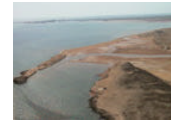
Djibouti site under development
